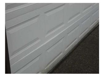
**46. Improvement Item :>** Only one of the overhead garage doors has an automatic opener installed. Installation of an additional opener may be desired depending on your plans for the garage.
