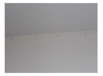
**48. Repair :>** Cracks were noted in the sheetrock ceiling of the garage. These are following sheetrock seams and appears to be poor workmanship. Implement repairs as desired and monitor.
