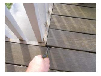
**43. Repair, WDO :>** Localized wood rot was noted in the railing system for the deck stairs and the handrail is damaged at the top landing - see how return is missing. The entire railing also needs to be painted and loose posts secured. Implement rot repairs and painting repairs to handrail system for this deck.
